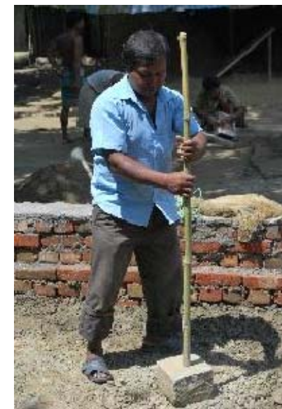
Compacting the plinth (taken from different house)
