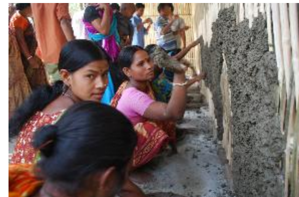
2 Workshop participants applying cement stabilised mud to walls
